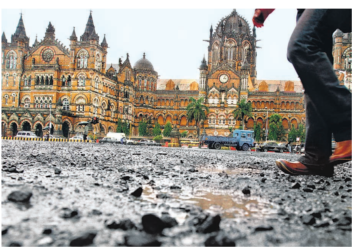
The pothole-ridden road right outside CST station, barely 30 metres away from the BMC headquarters, is an indicator that the municipal corporation has its work cut out trying to meet the August 30 deadline set by the high court to free the city of potholes. Clearly, the work will have to begin at home. But Municipal Commissioner Johny Joseph says the civic authority will undertake the task with zeal. "Potholes anywhere will be taken care of before the August 30 deadline," he told DNA on Thursday — Kamlesh Pednekar.DNA
